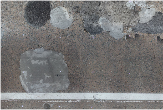
Fig. 13 Stitched image of a section of the Haymarket Bridge deck
